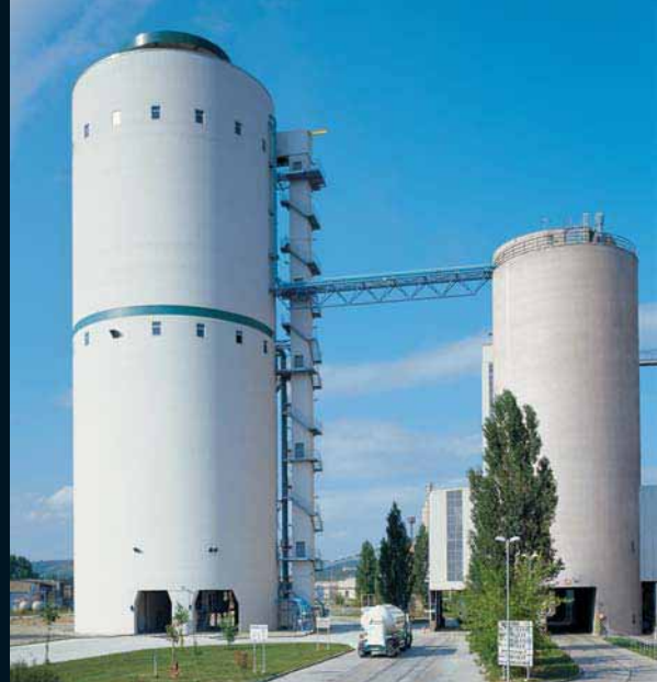
LAFARGE CEMENT, Karsdorf works, Germany
