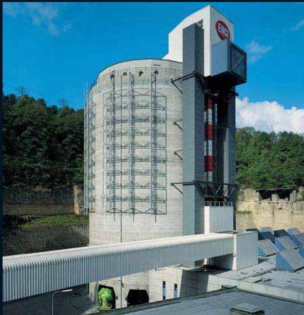
ENCLEERSTE NEDERLANDSE CEMENT INDUSTRIE Multi-Compartment Silo, Maastricht, the Netherlands
